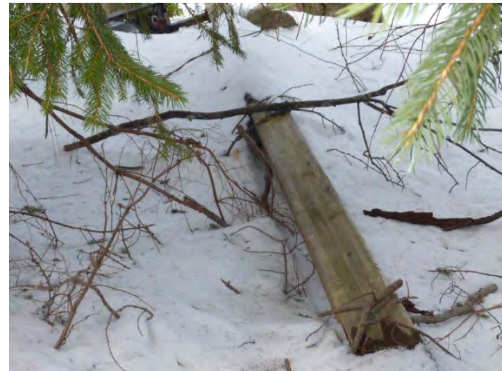
Light pole along drive has failed and collapsed. New poles are shown in Year 1 of the plan.
