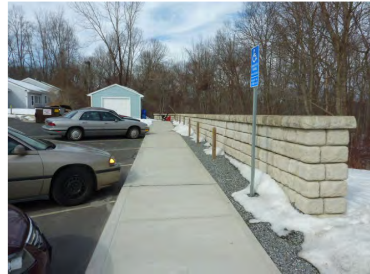
Typical concrete walk and curb along retaining wall and new parking.
