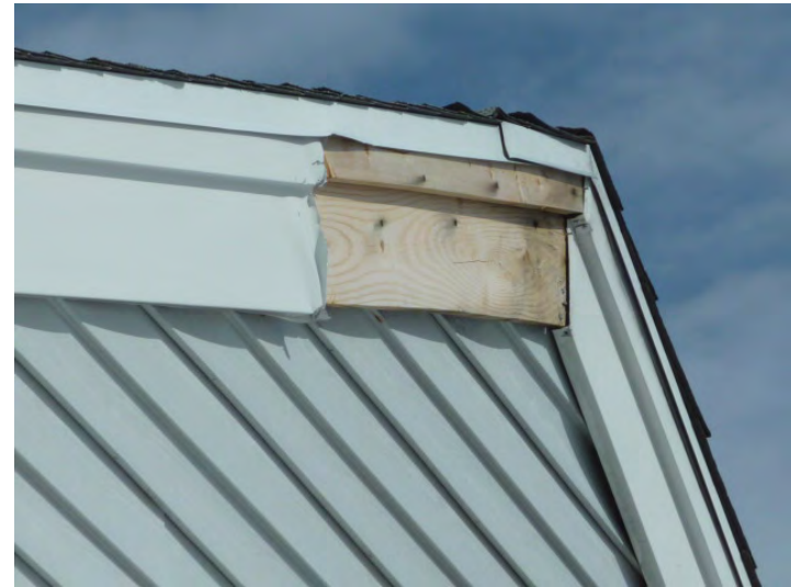
Storm damage at fascia at select locations.
