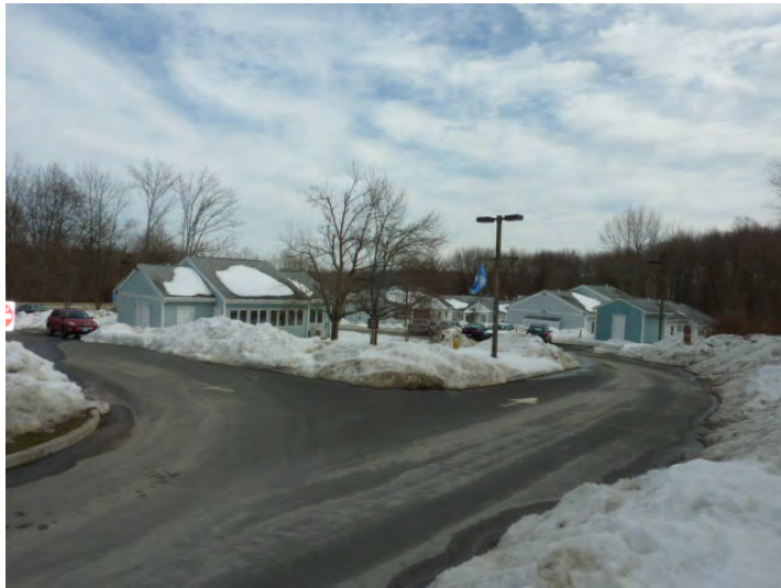
Asphalt drive at the Community Center and site-wide has concrete curb and is in good condition.
