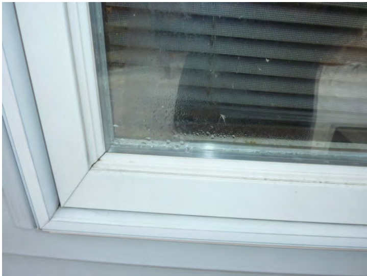
Typical failed insulating glass seal at windows.
