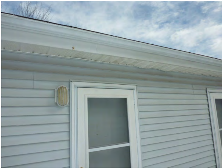
Typical soffit deformations at select locations.
