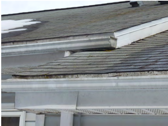
Worn and curling asphalt shingles.
